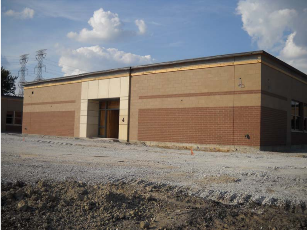
View of south façade.
